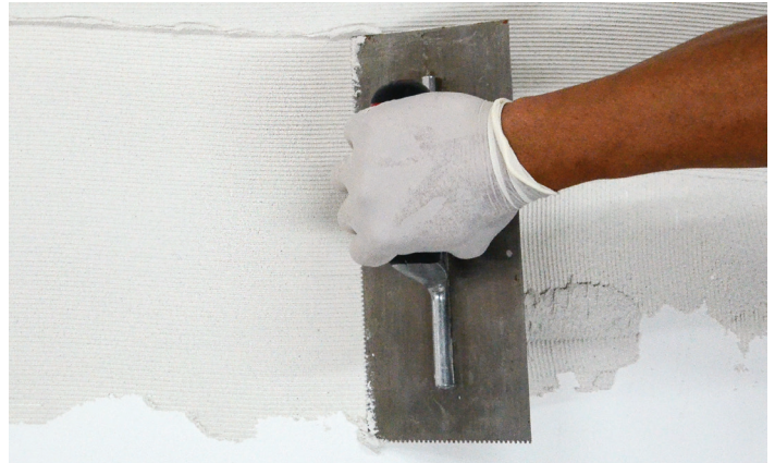
Step 2 To establish the proper depth of the setting bed, use a \frac{3}{16} " x \frac{1}{4} " v-notch trowel to apply additional thinset and comb full notches in one direction.
