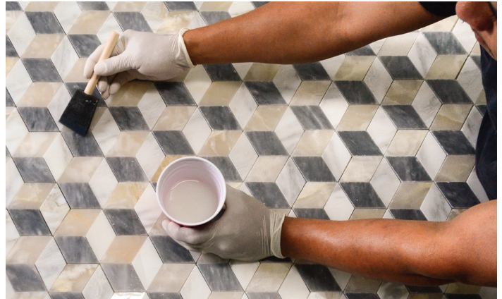
Step 6 Apply Oceancare penetrating sealer as grout releases, per manufacturer's instructions.
