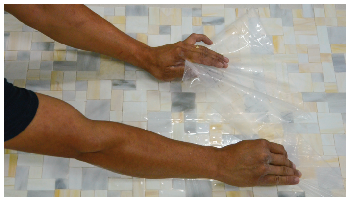
Step 6 After 24 hours of cure time, peel the tape from the tile starting from the corner. Use an angled downward movement.
