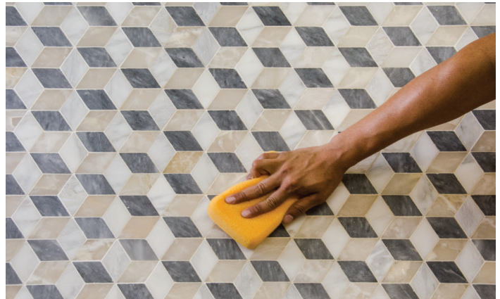
Step 9 Allow grout to set until firm and smooth finish with a damp sponge. After approximately 2 hours, remove grout haze with a lightly damp sponge.
