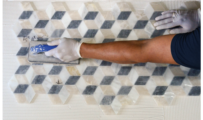
Step 4 To achieve the flattest possible surface, lightly tap the sheets using light pressure with a grout float or a wooden beating block and a finish hammer. To unify sheet transitions, tap from one sheet to the next.
