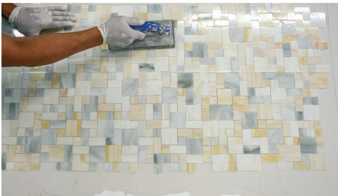
Step 5 To achieve the flattest possible surface, lightly tap the sheets using light pressure with a grout float or a wooden beating block and a finish hammer. To unify sheet transitions, tap from one sheet to the next.
