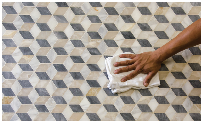
Step 10 For final removal of grout haze, polish with a clean, soft, white cloth.
