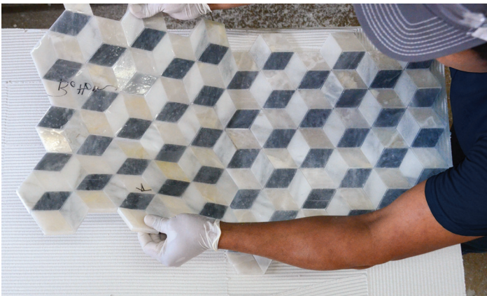
Step 3 Apply mosaic sheets to the thinset setting bed, tape side toward you, with light, even pressure. Periodically, check thinset for skinning (slight drying). If skinning occurs, remove thinset and reapply.
