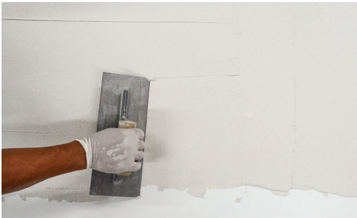
Step 3 Use the flat side of the trowel to flatten the notches and achieve a smooth, consistent thinset setting bed.
